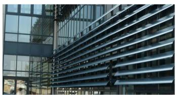
Figure 17. Movable horizontal aluminium sun shading elements proposed to be applied on the south facade of the building [26]
